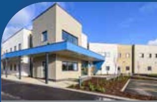
Cygnet Hospital Sherwood, Nottinghamshire
